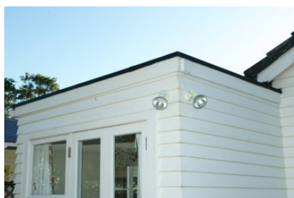
Figure 4: Bitumen membrane skillion roof
