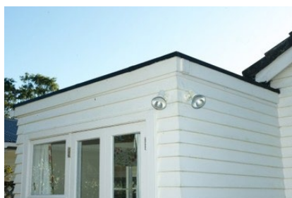
Figure 4: Bitumen membrane skillion roof
