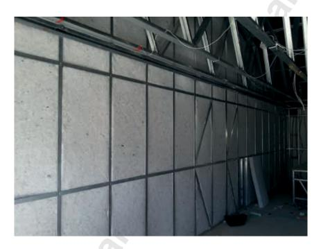
Figure 16 - Insulation fitted into a steel-framed wall
