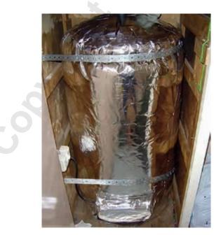
Figure 35 – Insulated hot water cylinder
