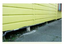
**Figure 7:** Areas of subfloor space with insufficient clearance
