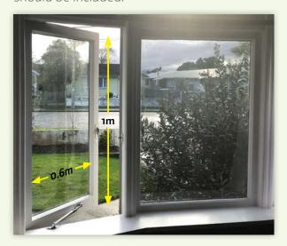
> multiply these measurements to reach a total openable area of windows, doors and skylights. Using the image above, the calculation would be 1 x 0.6 = 0.6. Record this figure (0.6) = Y.
